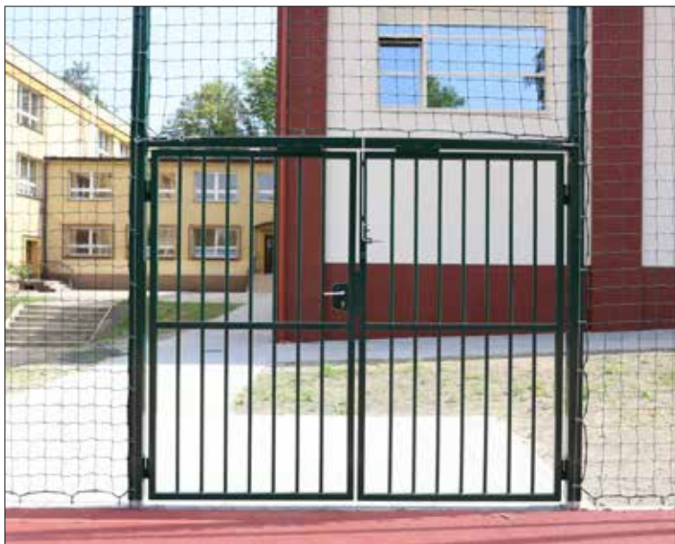
Steel fence between the posts of protection set
