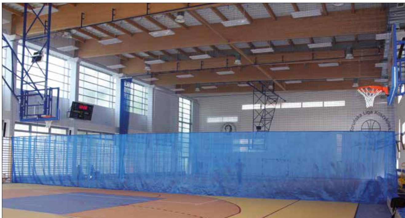
System for fixing and horizontal sliding of the curtain operated manually
