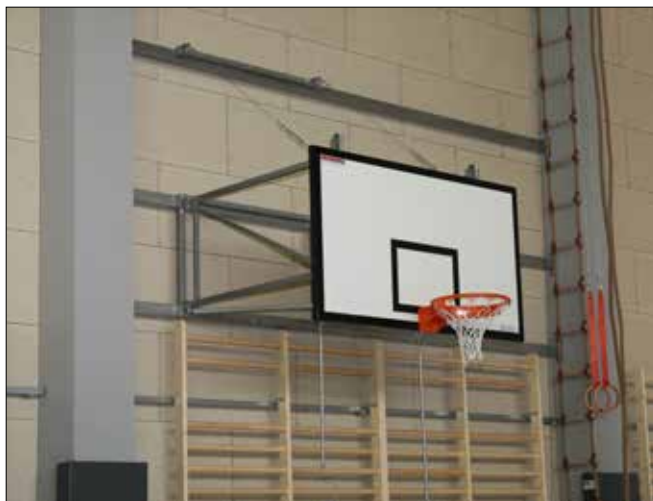
Structure mounted between reinforced concrete pillars
