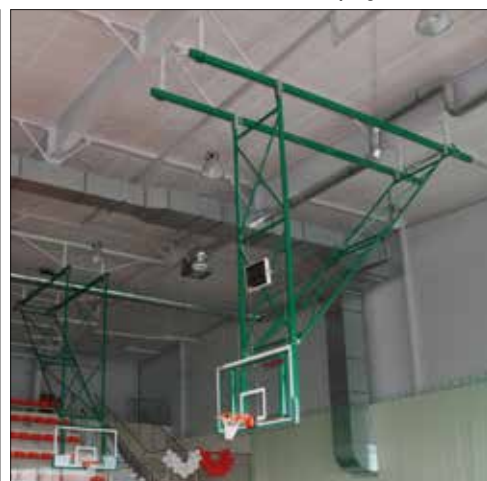
Mounting to a steel girder
