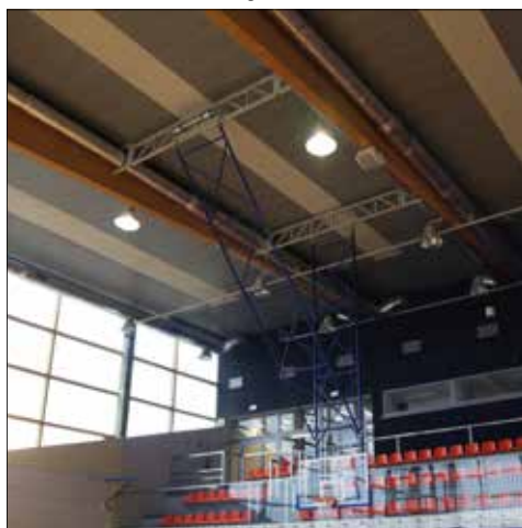
Structure mounted between girders
