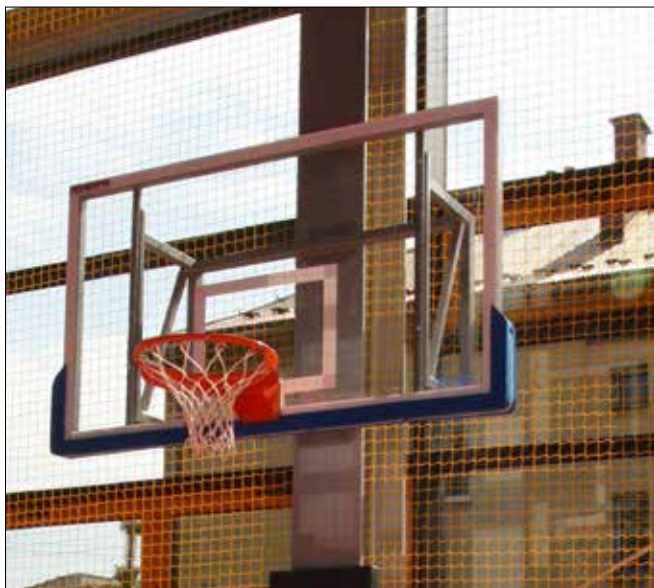
Structure mounted to the steel pillar
