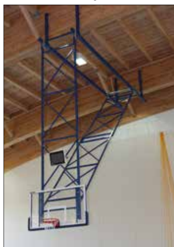
Mounting to a wooden girder
