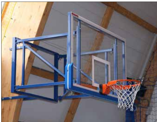
Structure mounted to a wooden girder
