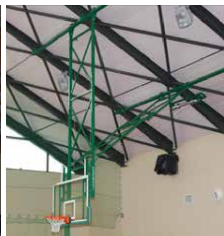
Structure fastened to the sloping roof
