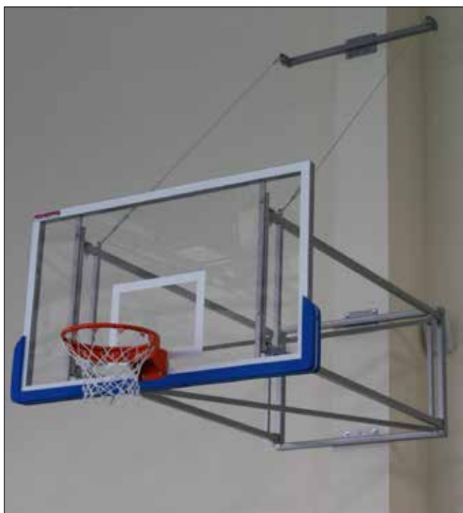
Structure mounted to the reinforced concrete pillar
